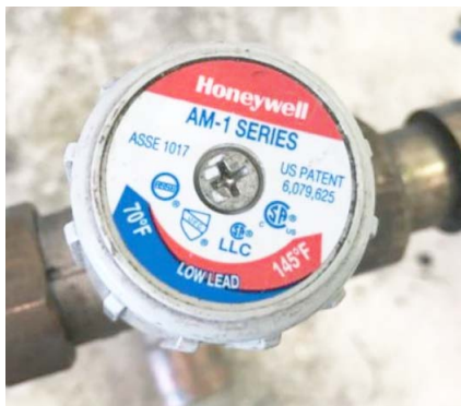
Hydronic Heating System Tempering Valve (Located below dinette seat - remove screws and panel to access)
